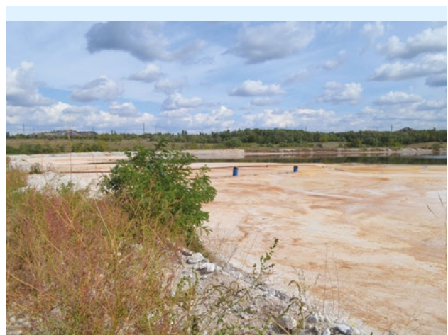
Figure 16. Formation of dry beaches at sludge SF No. 3 of the SMA Inkor & Co
