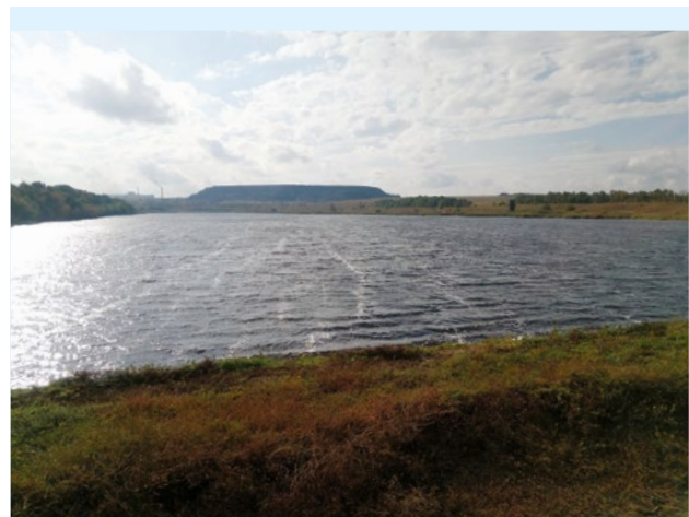
Figure 8. Storage pond, general view from the dam
