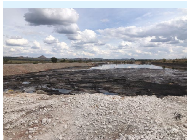
Figure 14. Sludge SF No. 1 of the SMA Inkor & Co
